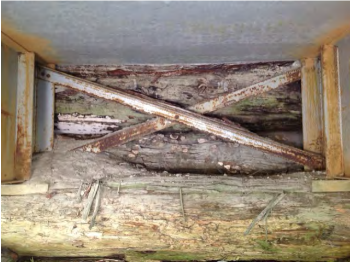
right abutment bracing condition
