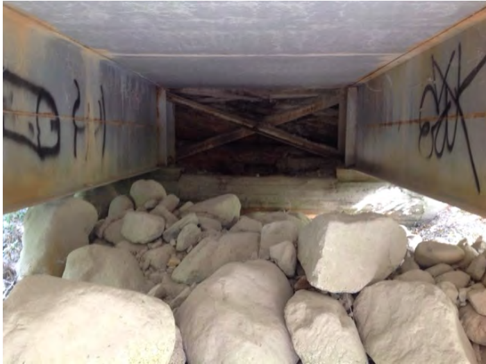
Left Bank Abutment when facing downstream
