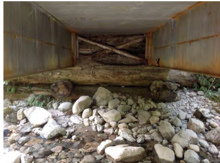
Right Bank Abutment when facing downstream
